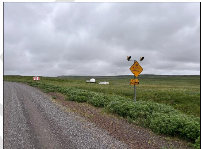
Enhanced roadway safety includes improved traffic control devices that utilize lighting and higher visibility signage.
