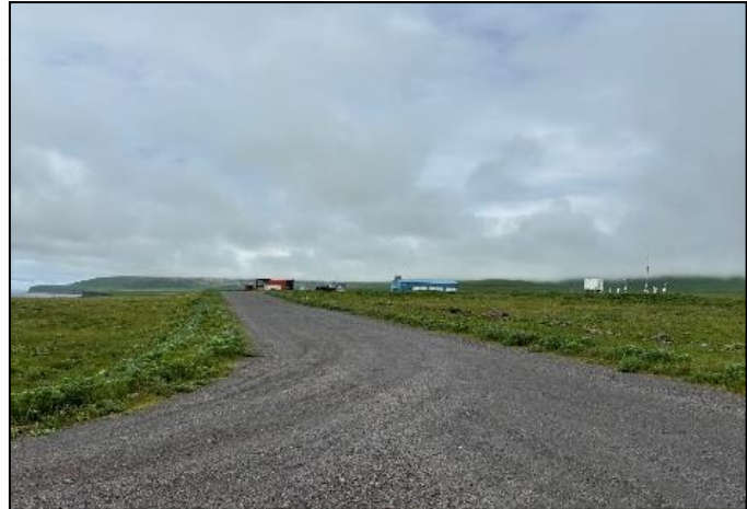
Saint George Island roadway developed using D1 gravel.
