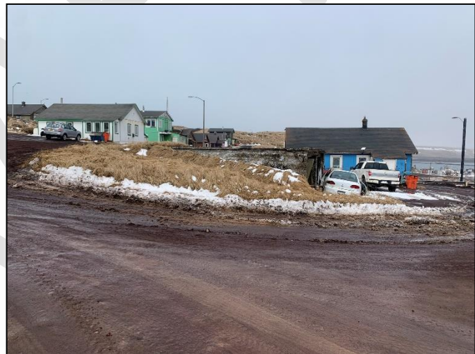
Saint Paul Island Community Roadway
