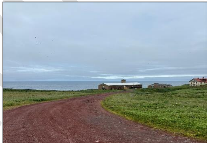
Saint George Island roadway developed using scoria rock.
